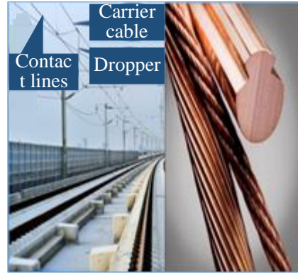
Fig .3. Bionic functional surfaces manufacturing Fig .4. High-speed railway contact lines with CuCrZr alloy
